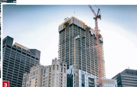
up to seven feet thick in places, with pipes and electrical conduits running through it, all modeled by computer ahead of time. That feature is necessary to distribute weight from residential floors above, which are held up by more columns than the office space below, said John Newhall, a project executive with Suffolk Construction.
